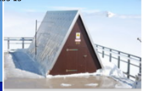
The housing of the Bonner Spheres Spectrometer including 16 Proportional Counters at 2650 m above sea level Germany
